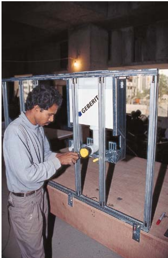
Prefabrication in the workshop
